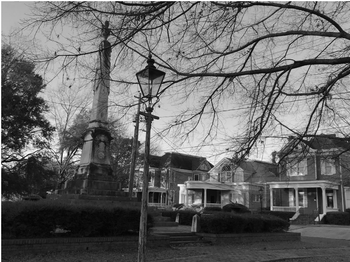
View of the monument showing its residential setting Photograph by Daniel A. Bellware
