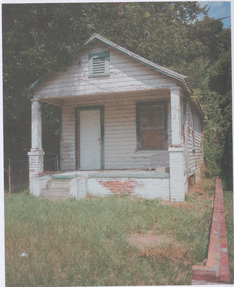
Boarded up Shotgun with Brick Wall on 10th Street, by Christopher Gass
