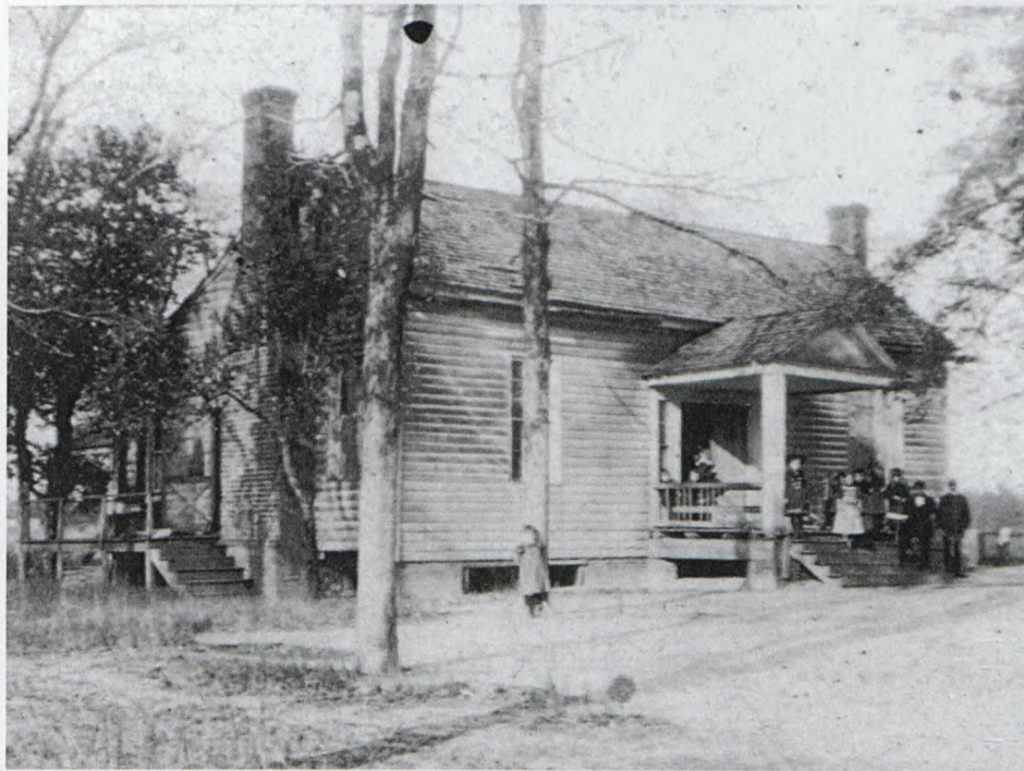
Fig. 15. Titled the "Elms," one of the most elaborate with two brick chimneys and what appear to be brick house footings.
